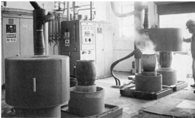
Fig. 6 Foundry installation of high-frequency induction lift swing furnaces.
